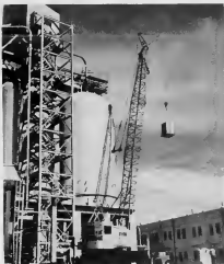
WHEN THE PCAR catalyst elevator failed recently, a crane was substituted to lift catalyst to hoppers. ORA CU e lift di catalyst a faya recientemente, un grua a worde substituí pa hiza catalyst pa hoppers.
